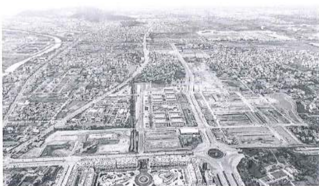
Overview of the project under construction
