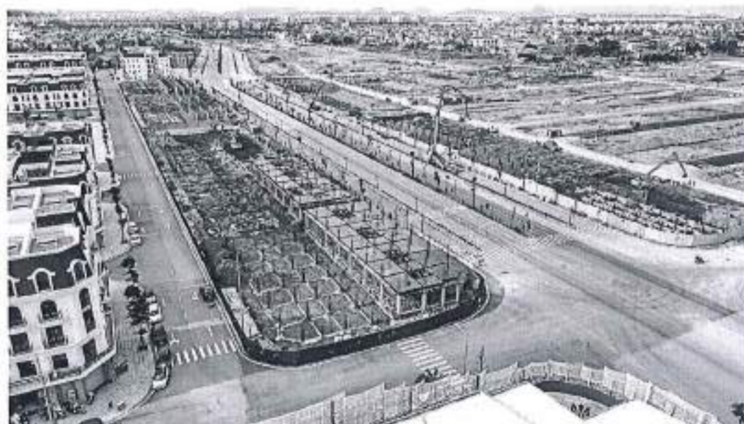
A corner of the project is implementing the construction of internal infrastructure, building a number of adjacent housing areas as of June 2025.
